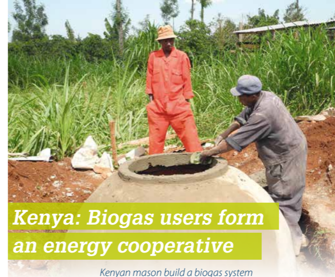
Kenyan mason build a biogas system
