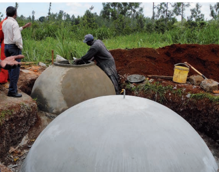
Building a biogas system in Kenya
