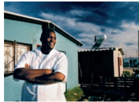
Kuyasa: Solar collector on roof
