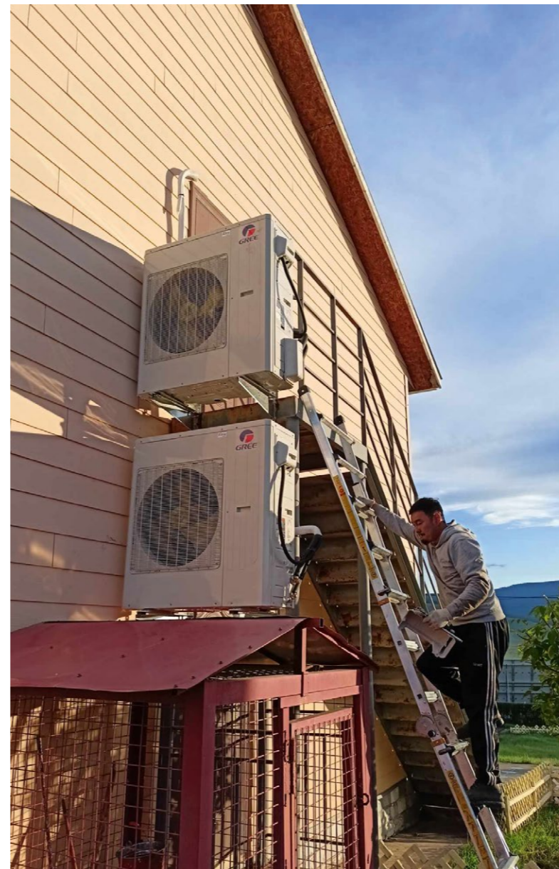
A worker installs air conditioning systems at a school in Mongolia
