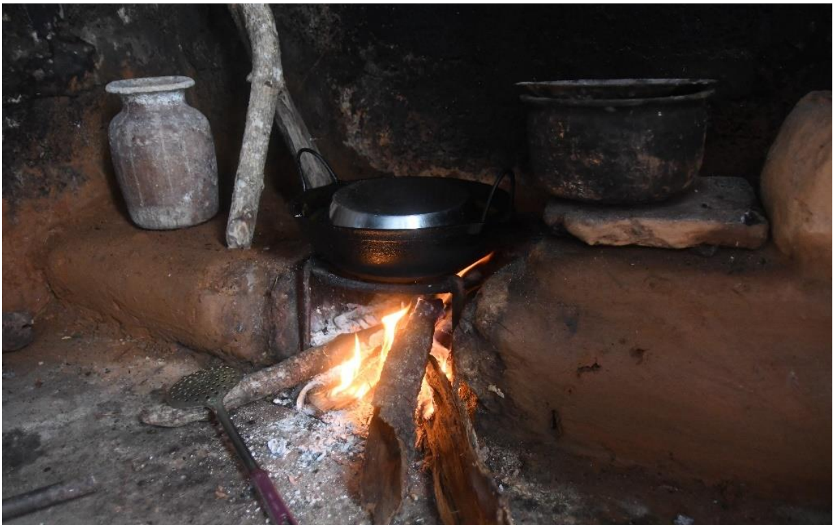
Picture 5: Due to the defective biogas plant, the family has temporarily switched back to firewood
