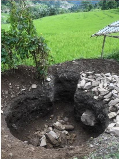
Picture 3: Civil engineering work for new biogas plant
